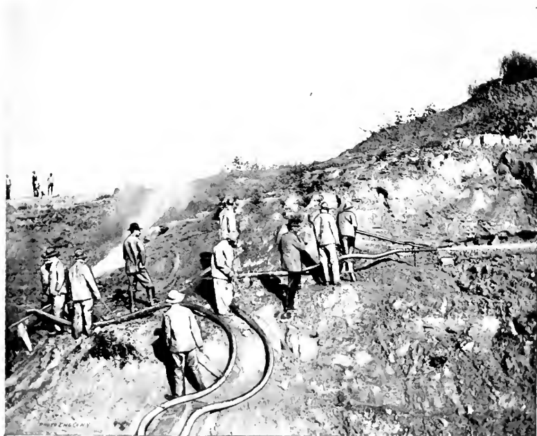
DETAILS OF HYDRAULIC GRADING.
